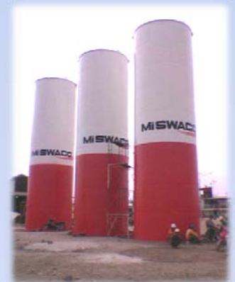
75m 3 Storage Tanks
